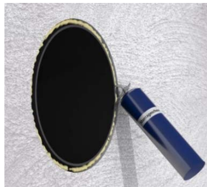
Fig. 5 Sealing the wall mounting pipe
